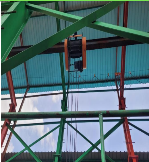
Machine used for loading & unloading of Raw Material into Tank
